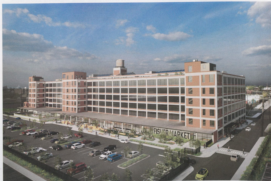
Fisher 21 Lofts will preserve the structure and features of the original 1919 Albert Kahn design including its window walls.
