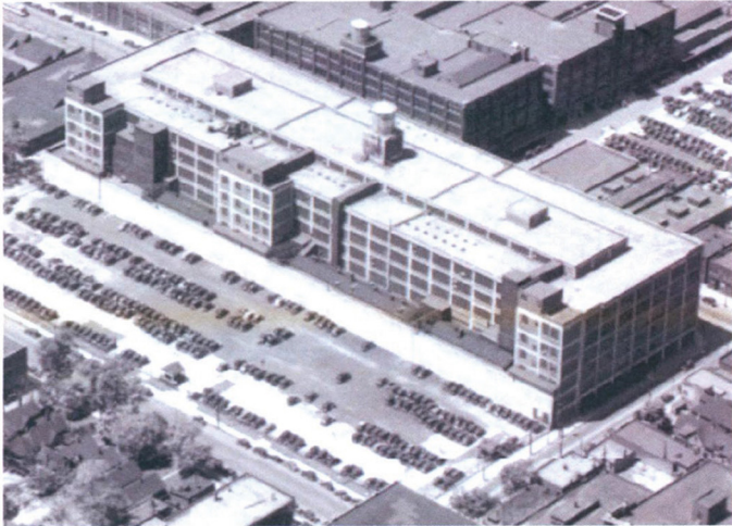
An aerial view shows how the Fisher Body 21 plant looked in 1936 when it was thriving by doing body and chassis work for General Motors.
